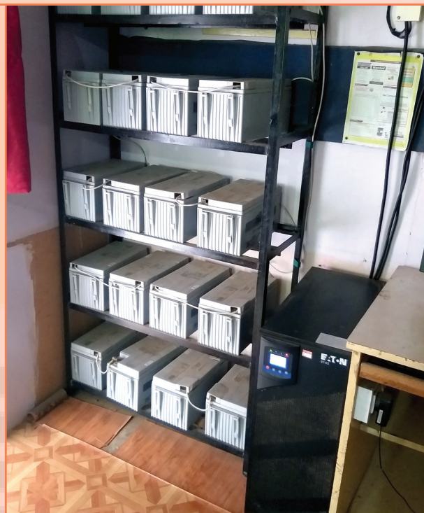
Solar operated battery inverter setup for Computer Lab at Bhairavnath Vidyalaya, Donde, Pune. Estimated No. of beneficiaries covered - 310
